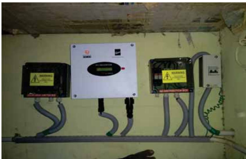
Figure 6 DCDB, ACDB, and 2 kVA inverter
