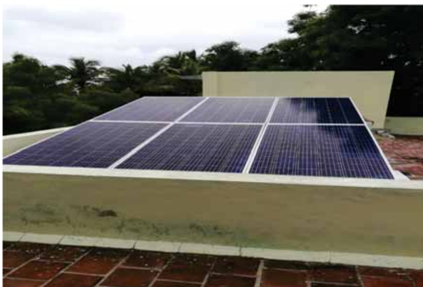
Figure 7 A 2 kW solar rooftop plant
